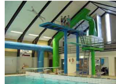
The swimming hall has just been renovated
